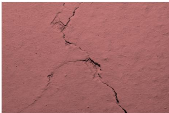
(a1) Original image of irregular network crack
