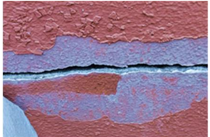
(b1) Original image of horizontal through crack
